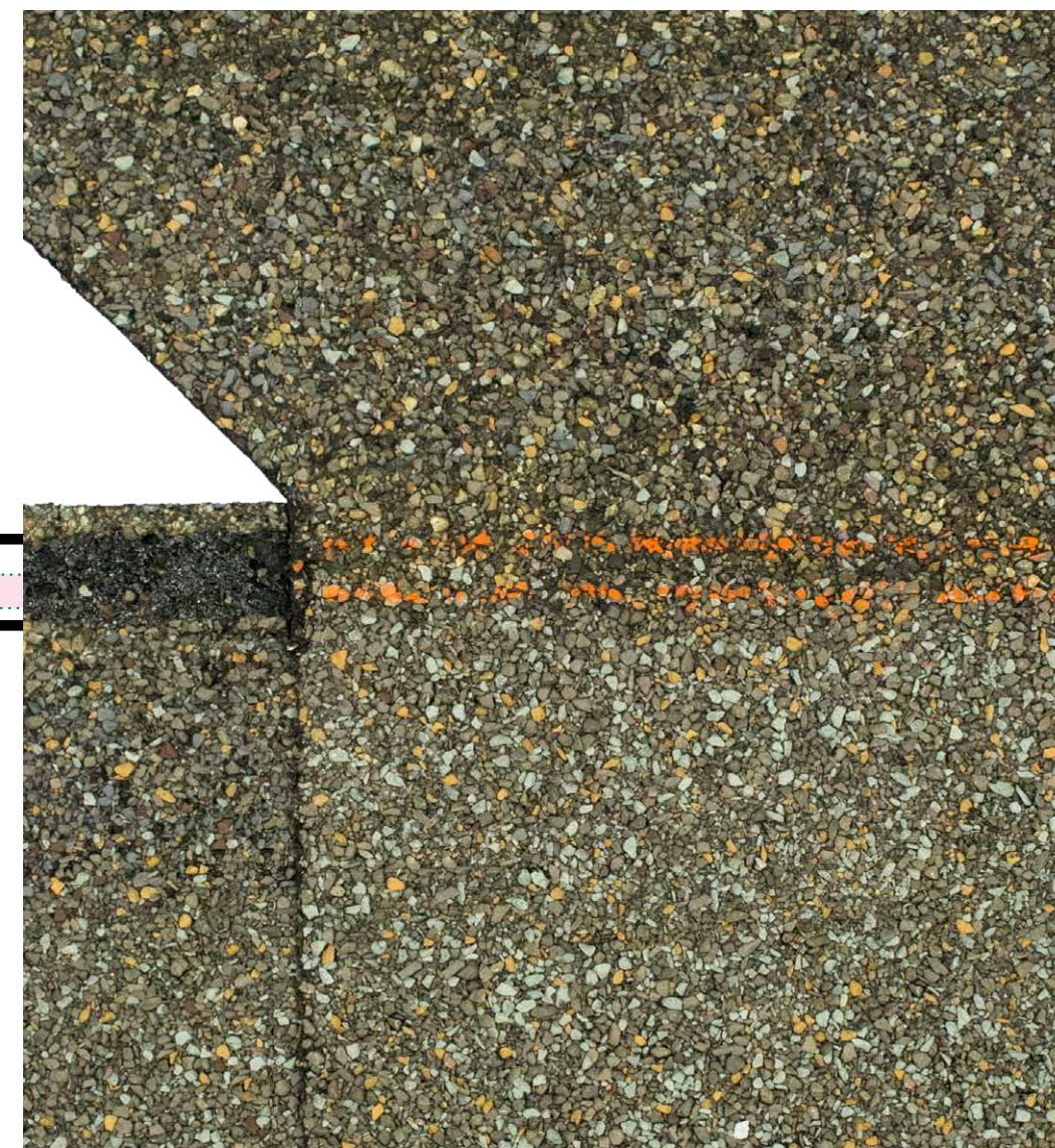
Standard Shingle Nailing Area - [1/2" to 3/4" wide, 1 rain seal]
