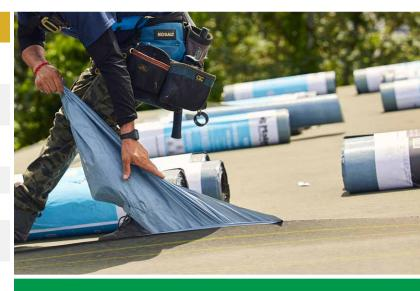
Easy-to-install roll assembly provides waterproof protection and meets UL 2218 Class 4 impact resistant standards when used as a system.
