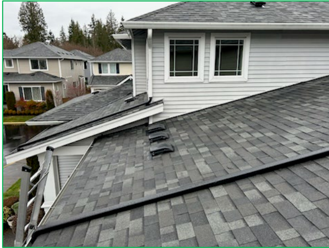
Examples of Enclosed Drainage Troughs: Connected to a Downspout (right); and Emptying into a Gutter Below (left)
