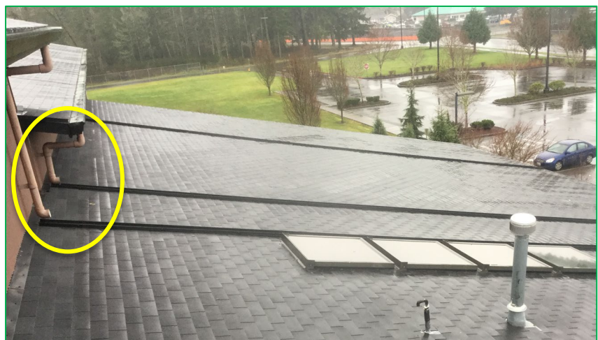
Examples of Open Drainage Troughs
