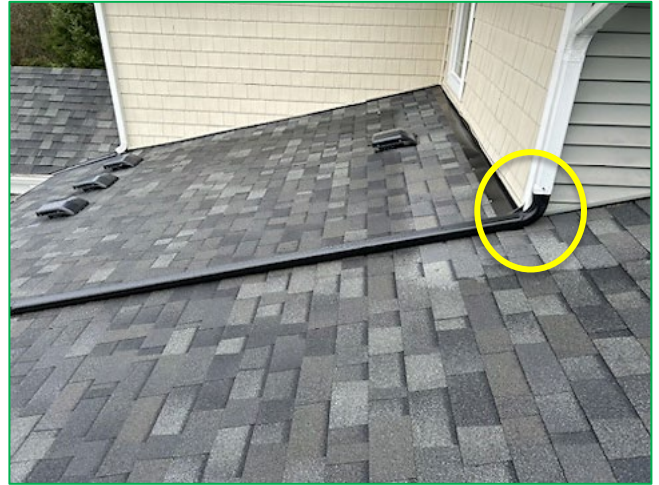
Examples of Enclosed Drainage Troughs: Connected to a Downspout (right); and Emptying into a Gutter Below (left)
