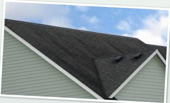
The picture below shows a roof in Florida after a 6-year period: shingles on the left have a 0% blend of copper granules while the right side has a minimum of 10%. Although results may vary based on climatic conditions, the difference in appearance is a dramatic and powerful example how shingles featuring Scotchgard™ Protector can preserve your investment by helping prevent black streaks on shingles caused by algae.
